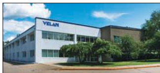
Williston, VT, U.S.A. Velan Valve Corp., Plant 3
