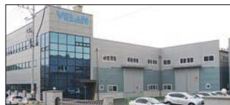
Ansan City, South Korea Velan Ltd., Plant 3
