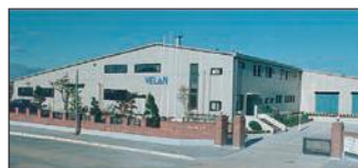
Ansan City, South Korea Velan Ltd., Plant 1
