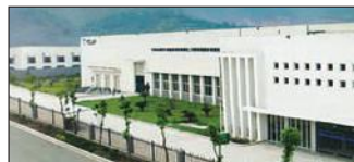
Suzhou, China Velan Valve (Suzhou) Co., Ltd.
