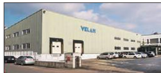
Ansan City, South Korea Velan Ltd., Plant 2
