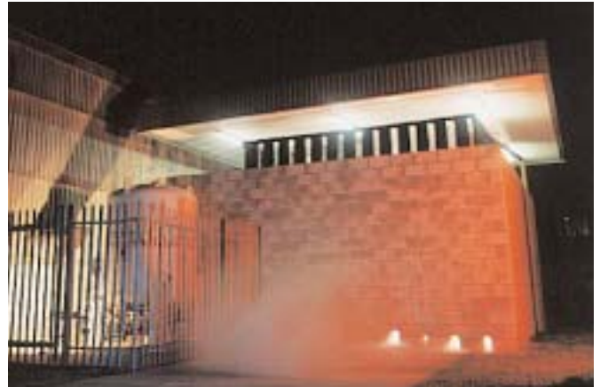
Cryogenic Test Facility/Explosion Proof Chamber.
