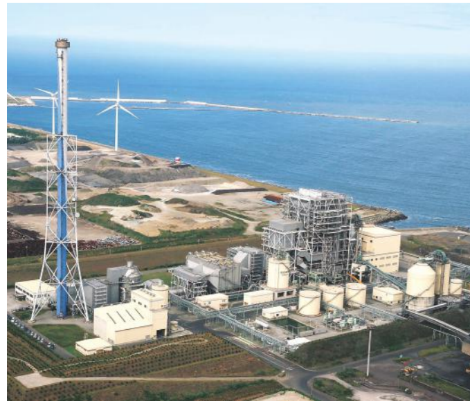
Appearance of thermal power generation boilers
