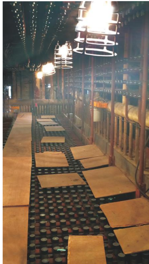
Inside view of a thermal power generation boiler under construction
