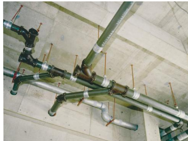
Various pipes in condominiums: ELP ® -NTA (gas, water supply, water drain, hot water supply, etc.)
