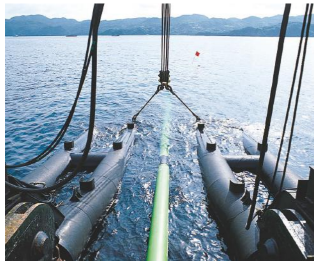
Offshore pipeline: NS-PEL ® (green)
