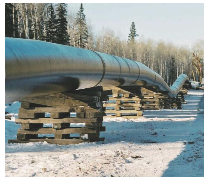
Installation of a pipeline
