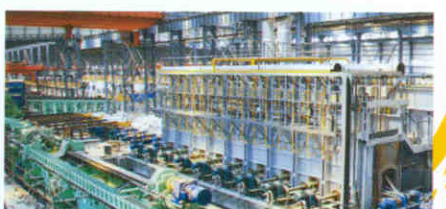
▶ 再加热炉 Heating furnace
