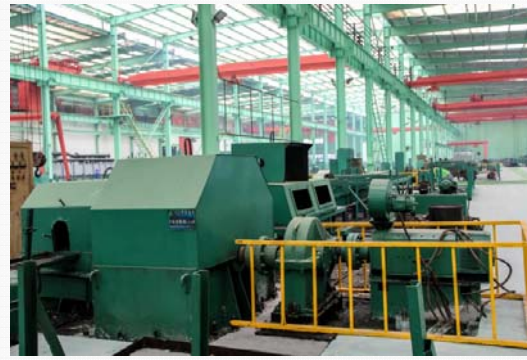
280mm Cold Rolling Produce Line
