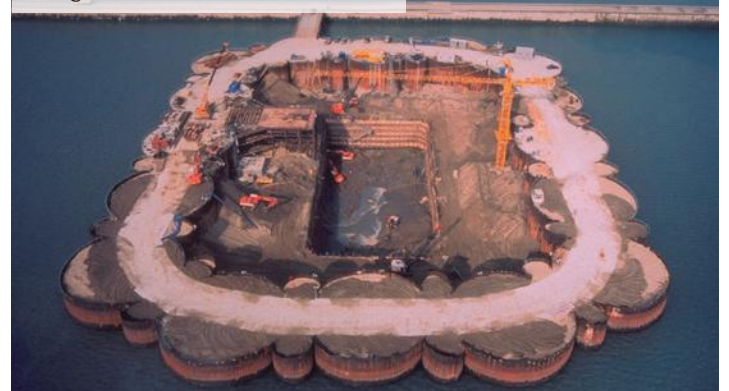
Bridge construction, South Korea
