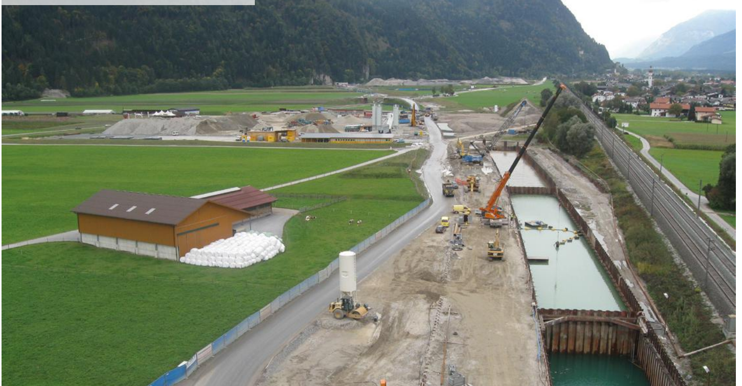
Temporary trench, Brenner railway, Austria
