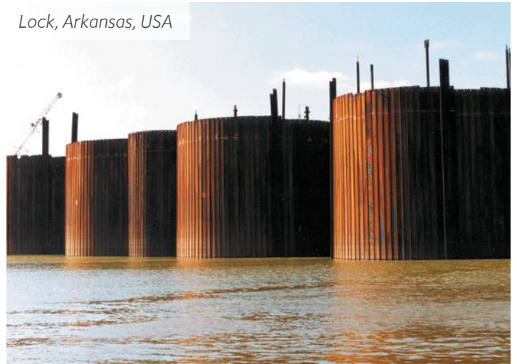
Diaphragm cells with 120^\circ junction piles.
