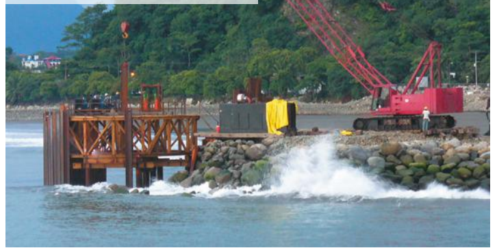
Marina breakwater, Costa Rica
