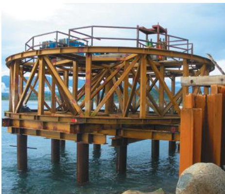
1. Installation of template
