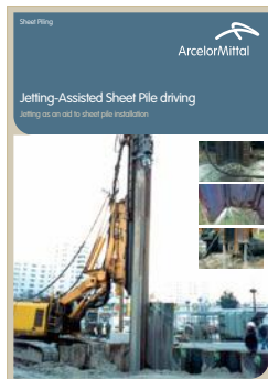
Jetting-assisted sheet pile driving GB, DE, FR
